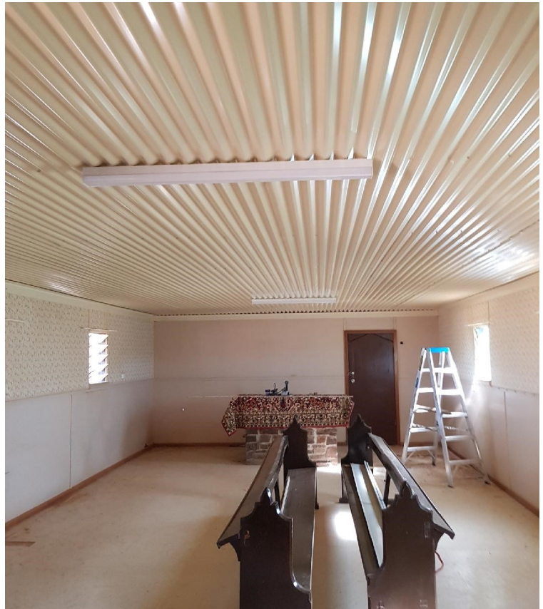
New ceiling and lighting has been installed.
