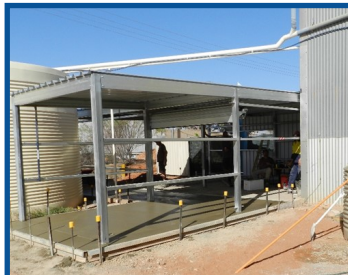
New secure store extension cement floor completed ready for cladding.
