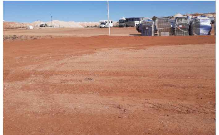
"Ground work in preparation for Pump Track installation."
