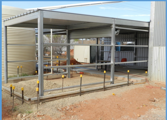
Taking shape. Note the servery and storage space with roller doors front and back.
