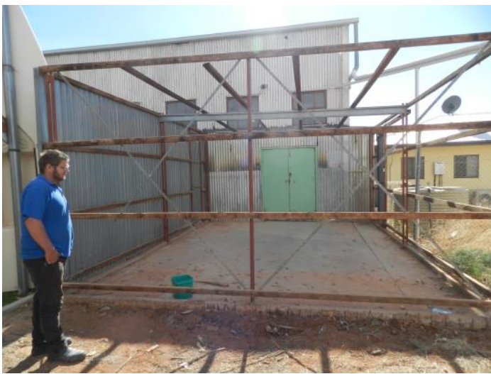
Moving forward with deconstruction of the leaky old store room. The old wooden framework will be replaced by metal and the structure will be enlarged by around 1m in length and 1.8m in width. The rear opens up into the community garden space and a side awning will open into the courtyard.
