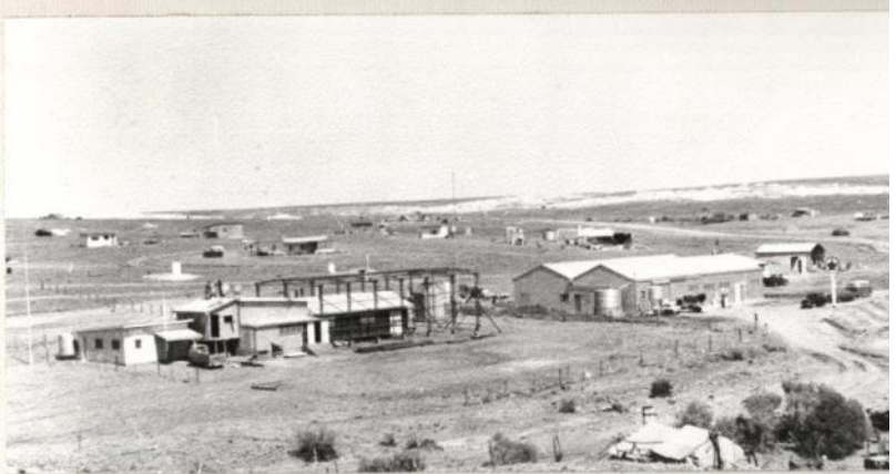
The framework of the 'new' hall going up over the old. The general store can be seen to the right of the structure. Photo: circa 1978.
