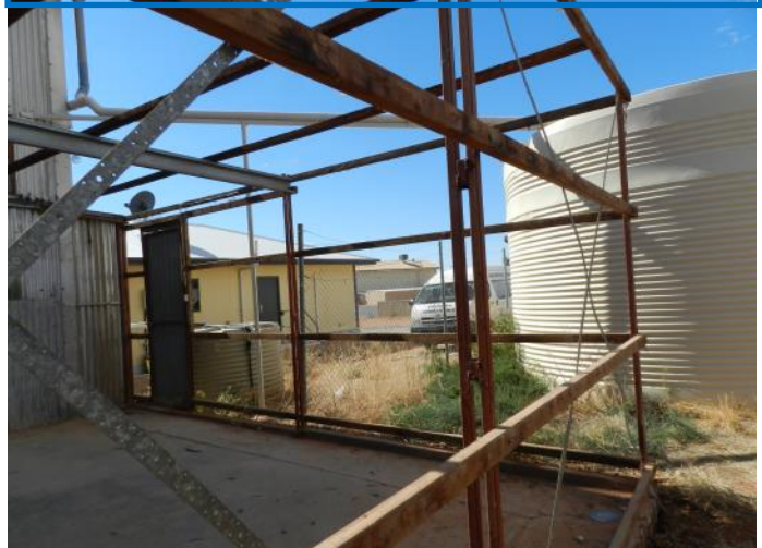
The image below provides a perspective to how a new storeroom will be constructed on the eastern wall from materials repurposed from the old storeroom and will extend into a carport to provide shade and undercover protection for the community bus. The small rainwater tank visible has been moved across and reconnected, just in time for the rain!
