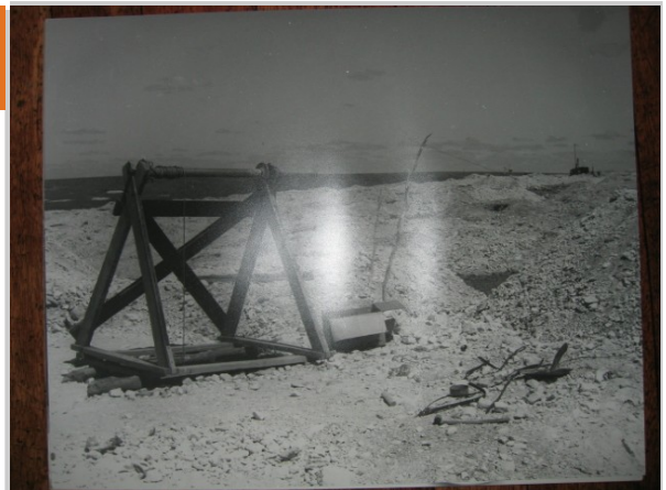
Early diggings with bucket & hand winch set up to hoist up the dirt dug in narrow underground tunnels by hand using picks and shovels .
