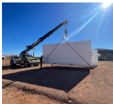
Above: New pad for the Community Produce Garden – April 2026
