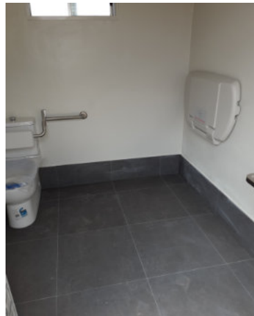
"Toilet block interior for Recreation Facility."
