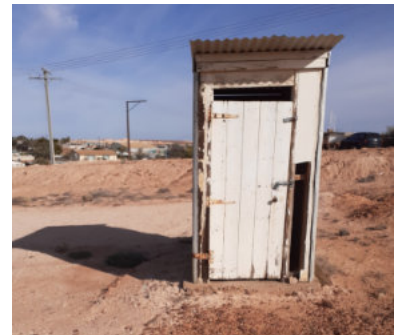
Existing toilet at the Community Church - To be replaced
