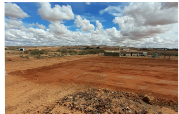
Ground work underway at new rec and sports centre!
